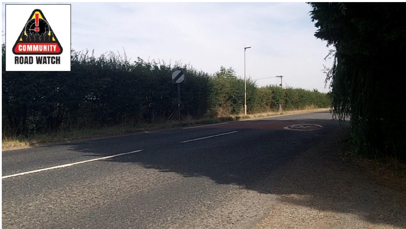
Willingham – Dangerous Overhang at Orchard Verge Cut Back so Children are safer
