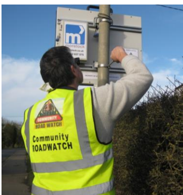
Andy Smith of CRW Installing the MVAS in Willingham
